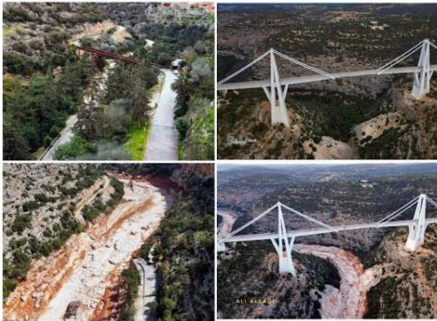
Figure 2. The catastrophic effect of Storm Daniel on Wadi Al kuf area from different locations. Left up, the wadi with the old bridge which established during Italian occupation before the flooding, and down, the devastation caused by the catastrophic flooding. Note the absence of the bridge, roads and vegetation. Right up the wadi new bridge. Note the differences between before flooding “up” and after flooding “down”. Photos were captured by the Libyan photographer Ali Al saadi (Al saadi, A., personal communication, October 10, 2023).
