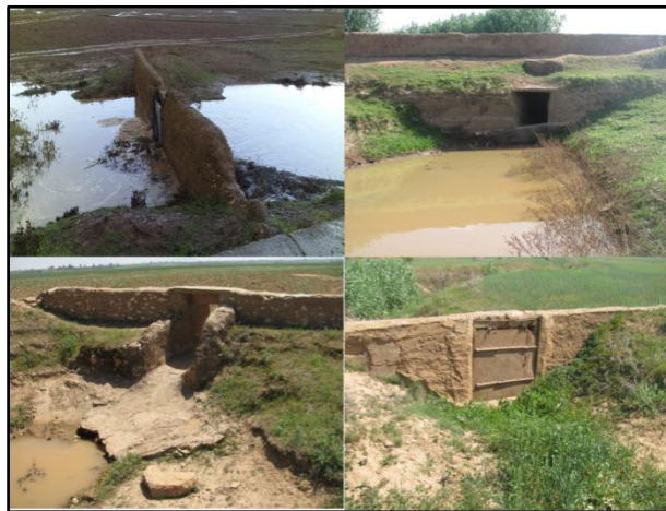
Figure. 7 Forms of the Rabta Technique
